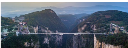
Walk Zhangjiajie's glass-bottom bridge
