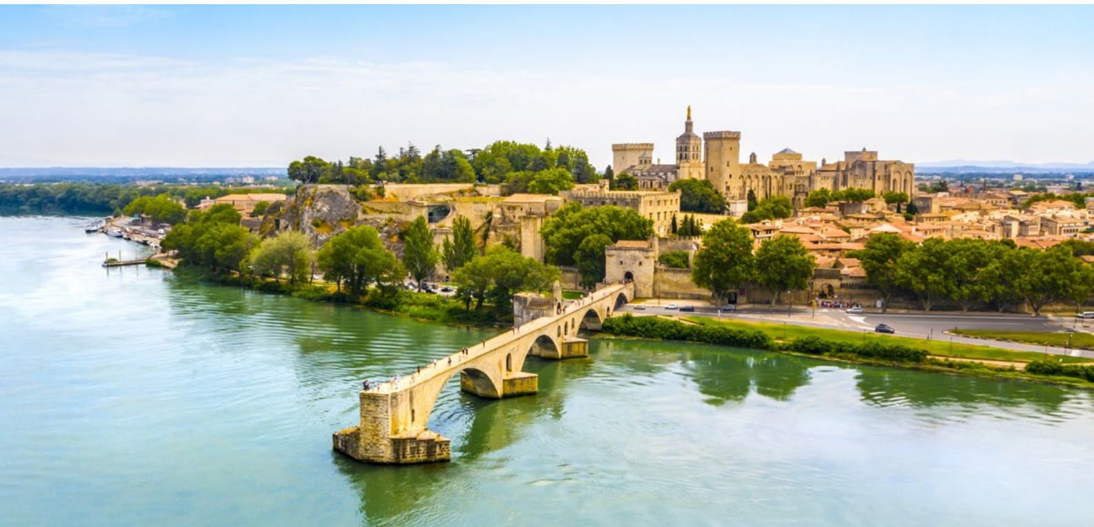
St Benezet Bridge, Avignon, France
