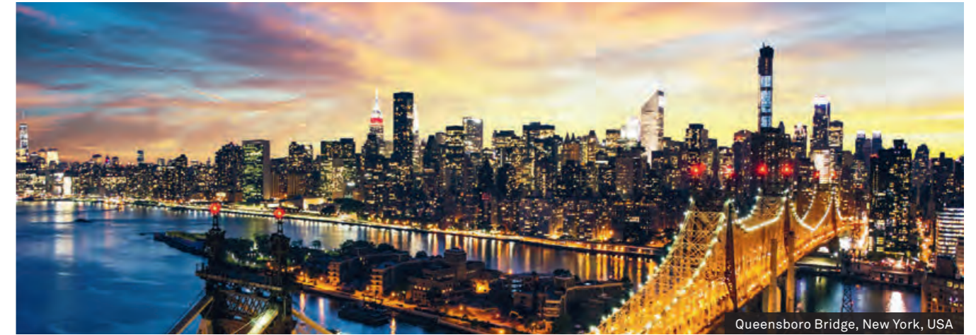
Queensboro Bridge, New York, USA
